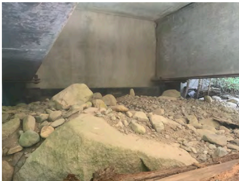
Left Bank Abutment when facing downstream
