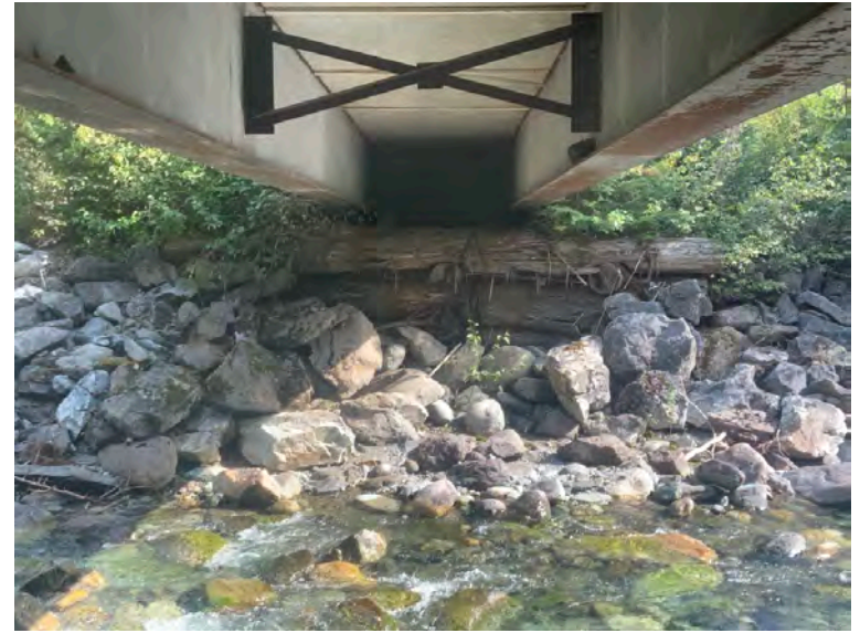
Left Bank Abutment when facing downstream
