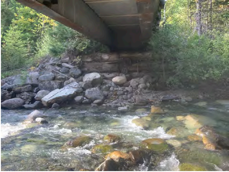
Right Bank Abutment when facing downstream
