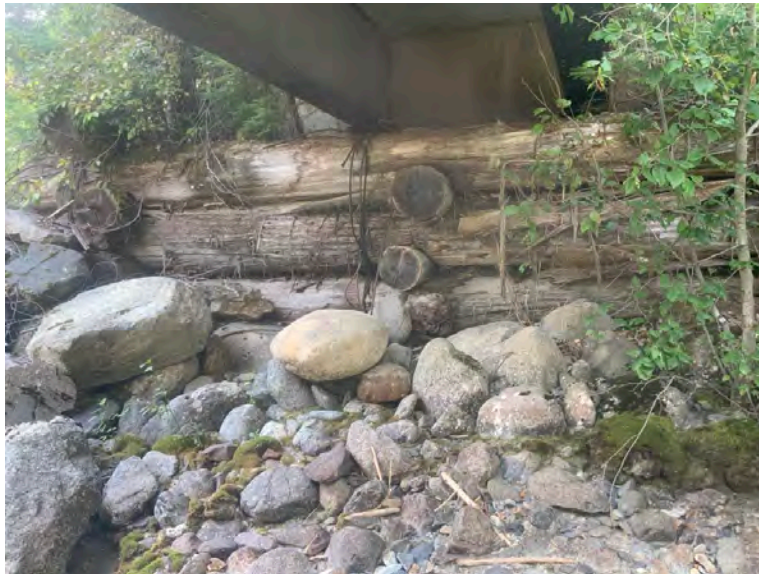
Right Bank Abutment when facing downstream
