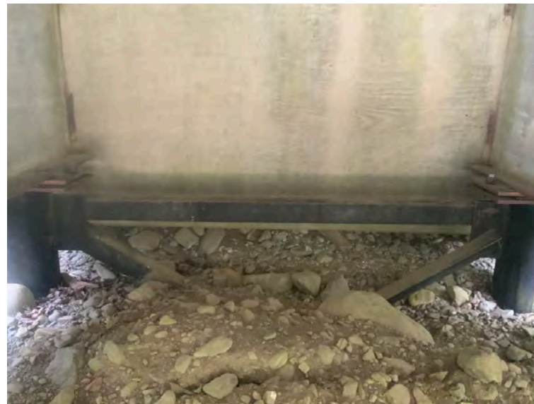
Left Bank Abutment when facing downstream
